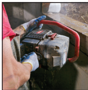
Safer to cut ductile iron
