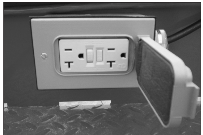
Figure 9.8 – Electrical Power Outlet
