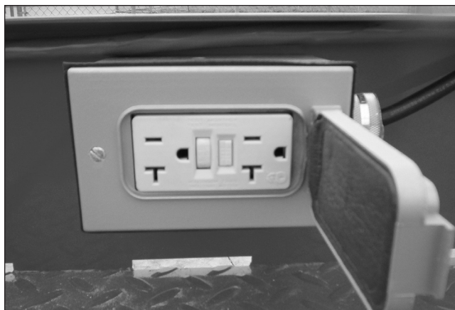
Figure 4.7 – Electrical Power Outlet
